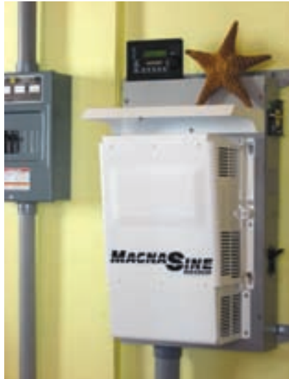
As the PV array expanded, so did the Barkers' power center. Although some of their primary loads are DC, three inverters (left and below) also convert the PV array's output for standard AC appliances.
