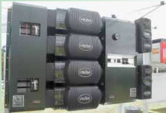
Shown here are four of Outback Power's FX inverters, their AC and DC boxes, and their MX-60 charge controller.
